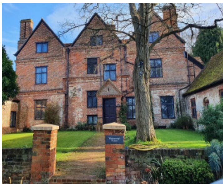
Wanborough Manor, Wanborough - 16th century (Grade II Listed)
