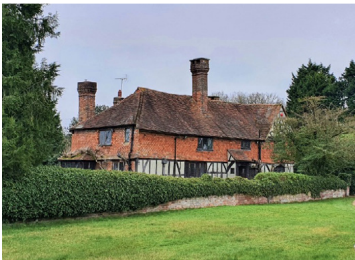
Traditional vernacular buildings on edge of Dunsfold
